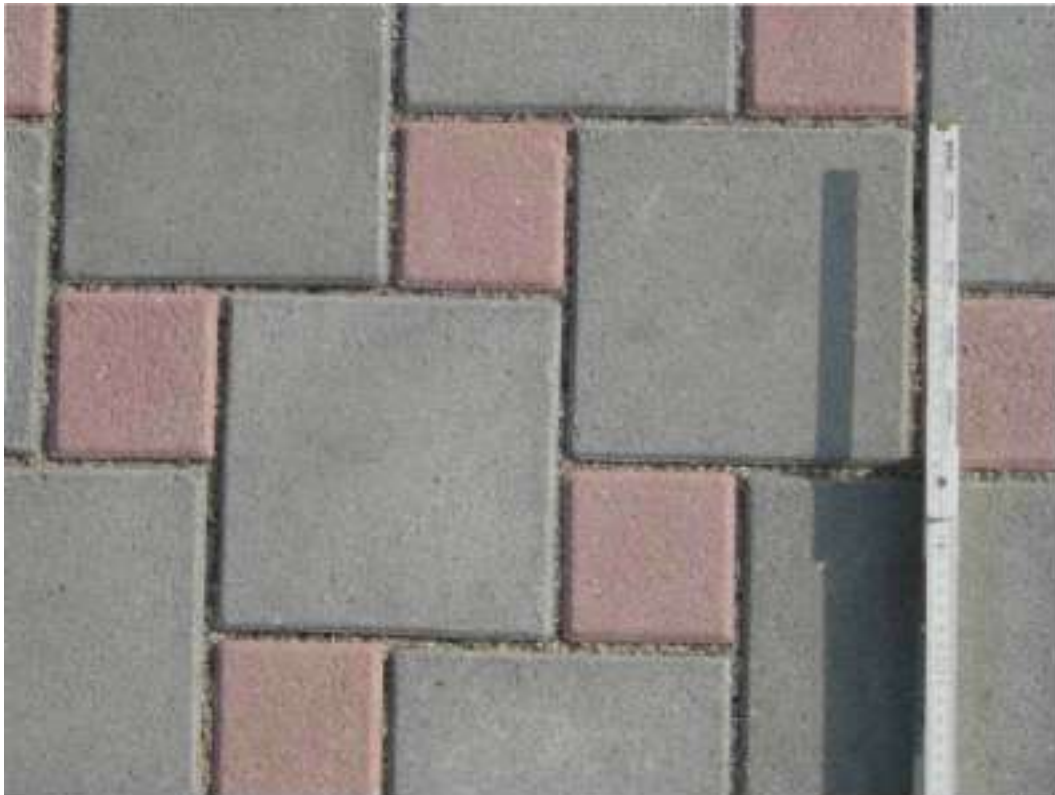
III. 1: PaVAge Pasero joints,5 mm pose canevas
